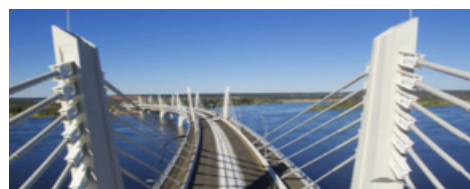
Kazungula bridge connecting Zambia and Botswana
